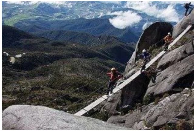
A suspension bridge between mountains.
